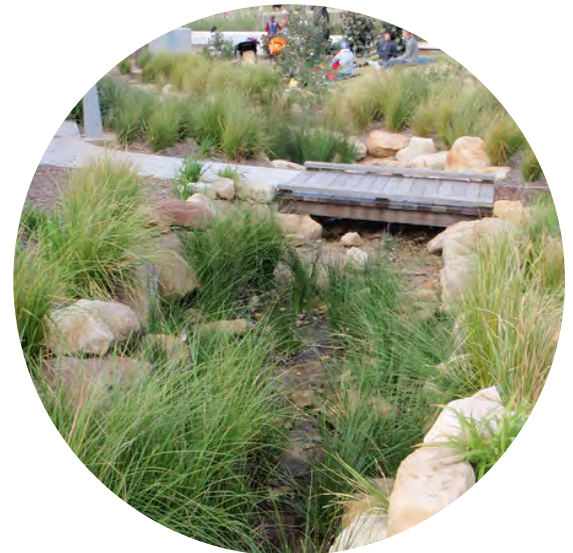
09 Bioswale with bridge crossing
